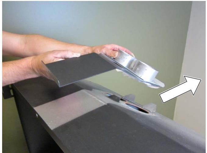
Connect the flex vent (exhaust and intake) to the vent connector (use self-drilling screws or hose clamps).
