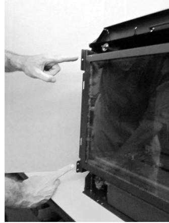
5. Attach the face bracket to the hinge bracket as shown below. The screws insert through the holes in both brackets.
