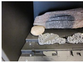
5. Place the #11 stone as shown below (the number is printed on the back of the stone). Note how the slot on the stone fits over the tab on the log support. **The printed number on the stone faces the rear of the firebox**.
