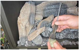
Apply a layer of rock wool over the burner ports.
