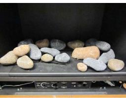
5. Place stone #16 at the left front of the firebox as shown below. This stone does not fit on a pin, but lies loosely on the burner.
