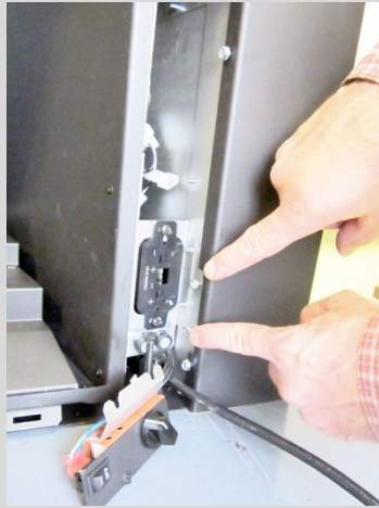
Install 2 screws (included with the insert) into these 2 penn studs. Leave a 1/4" gap.
