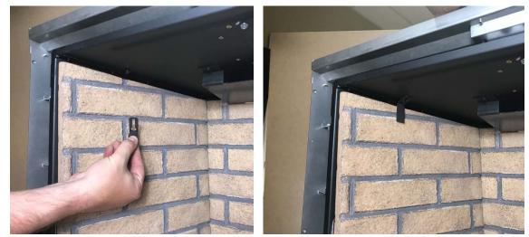
6. Install the right fireback and secure using the fireback clip. The firebox should now look like the photo below.
