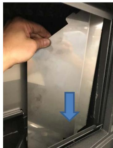
4. Tip the top edge of the side panel forward and guide the panel out of the firebox..
